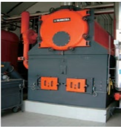
Figure 7 850kW biomass boiler for district heating application [10]
